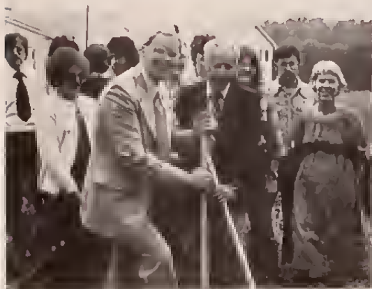
At ground breaking ceremonies for the new guest house, Dr. Bob Finley, left, and board member Walter Lumppp, right, begin excavation as staff missionaries look on. After the prayers were over, power shovels moved in to prepare the site for laying the foundation.
